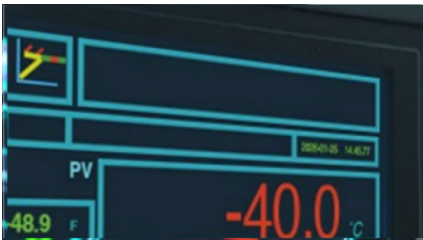
HMI Display: Low-Temperature Performance Test Under -40 °C
