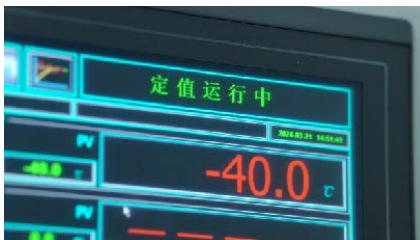
HMI DISPLAY: LOW-TEMPERATURE PERFORMANCE TEST UNDER -40°C
